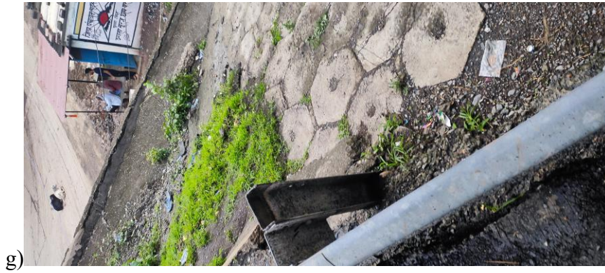
Figure 1 Observations: a-b) signs of settlement at embankment km 108+945; c-d) slope failure at embankment km 118+650; e-f) slope failure at embankment km 118+650; g) signs of surficial slope settlement and failure at embankment km 123+050
